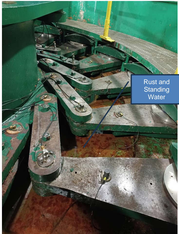
Figure 3-39: Head Cover from Turbine Pit
