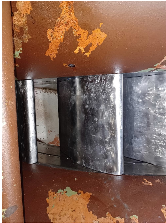
Photo 3: Wicket Gates and Stay Ring
