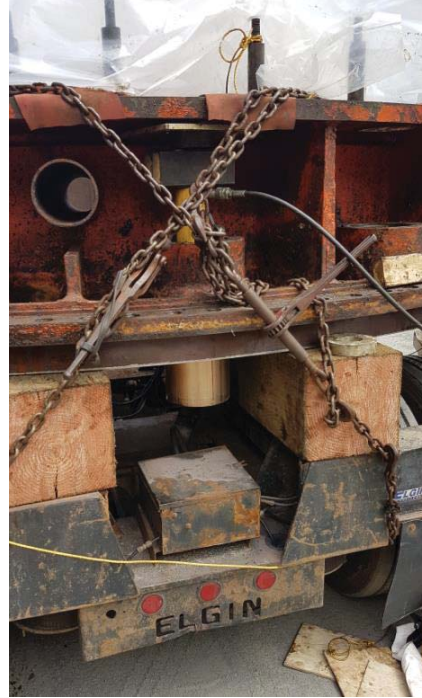
Figure 5-206: Head Cover, Intermediate Gate Stem Bushing Removal
