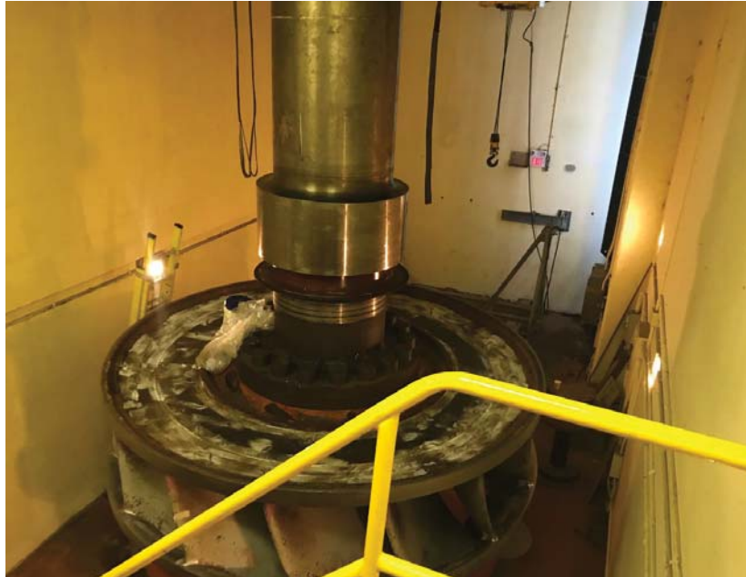
Figure 5-42: Lead Abatement (White Paste on Crown)
