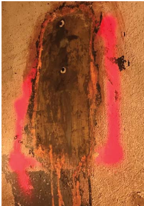
Figure 5-11: Draft Tube Void Mapping
