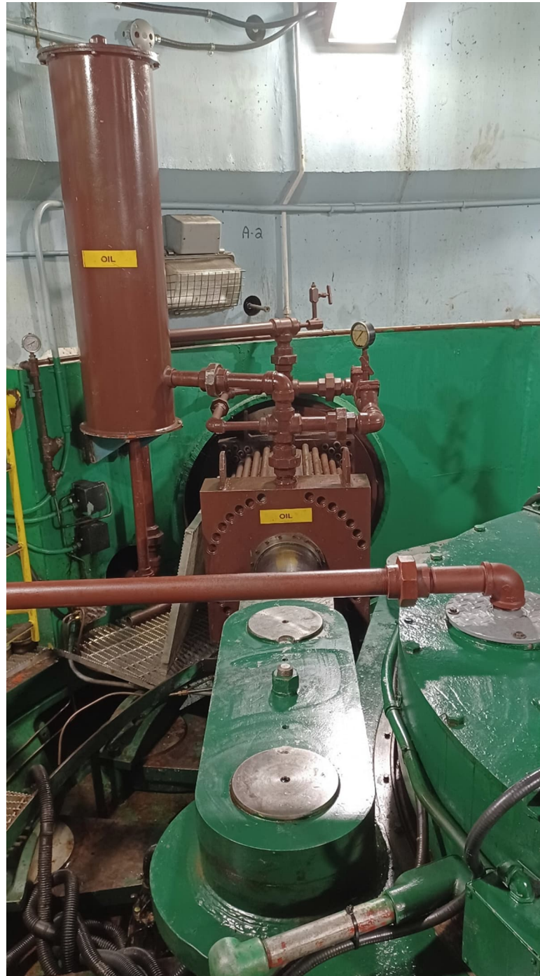
Photo 2: Dashpot in Turbine Pit
