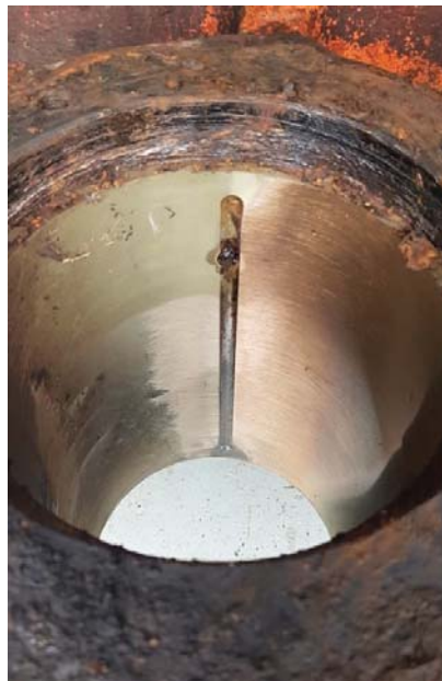
Figure 5-207: Head Cover, Intermediate Gate Stem Bushings
