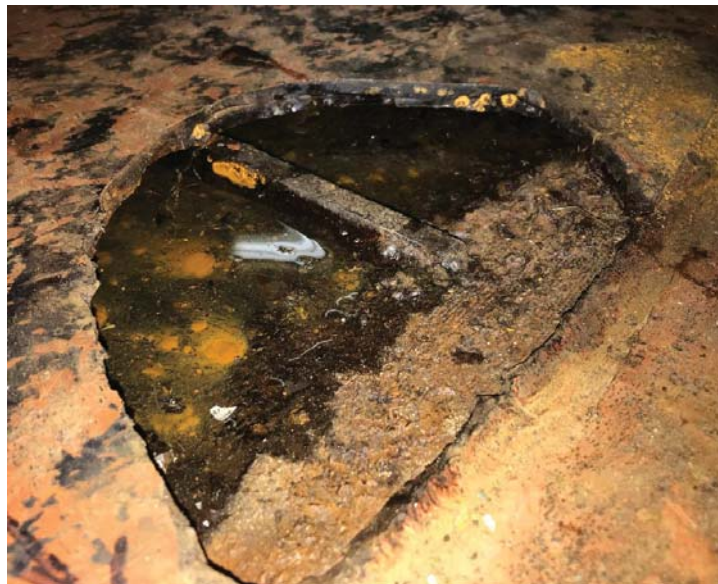
Figure 5-215: Runner Cover Balance Plate, Piece Missing
