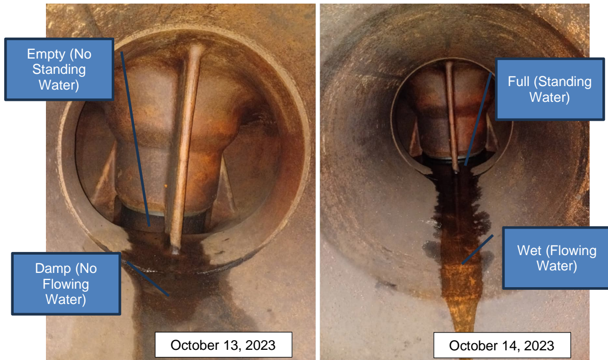
Figure 3-36: Leakage in Relief Valve as Seen from the Spiral Case
