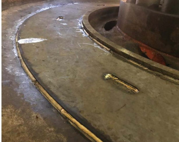
Figure 5-44: Runner Balance Cover Plate Repaired
