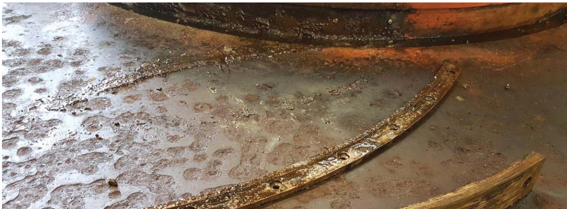
Figure 5-199: Head Cover, Paint Condition and Pitting of Upper Surface
