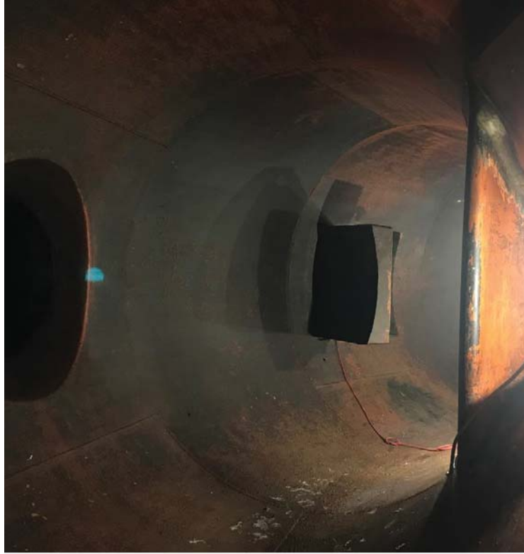
Figure 5-166: Spiral Case (Man-Door, and Pressure Relief Valve)
