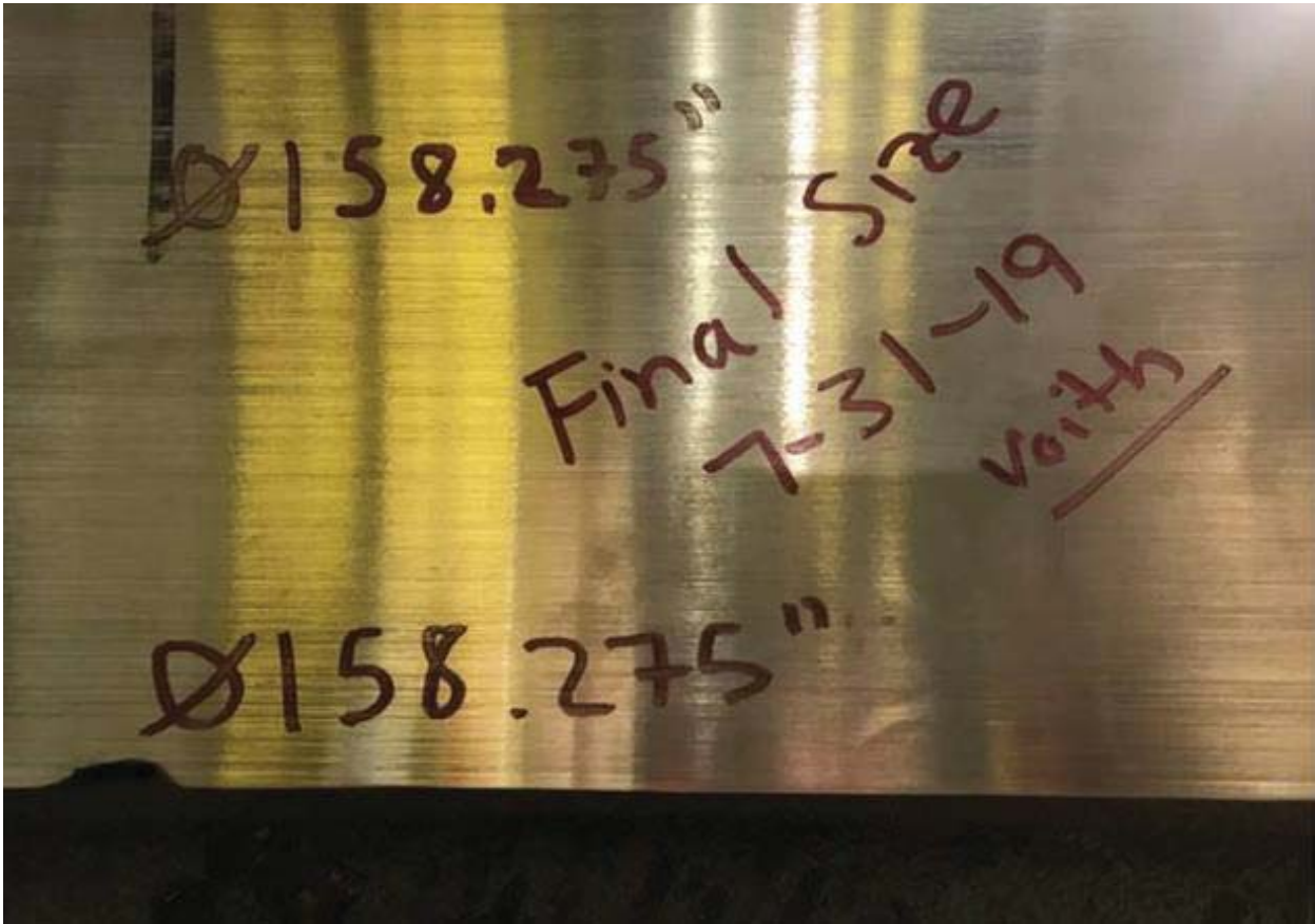
Figure 5-285: Final Bottom Ring Wearing Dimension – (Two Location)
