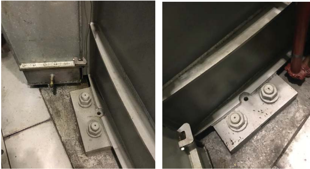
Figure 5-125: Stator: Stator Frame Sole Plates
