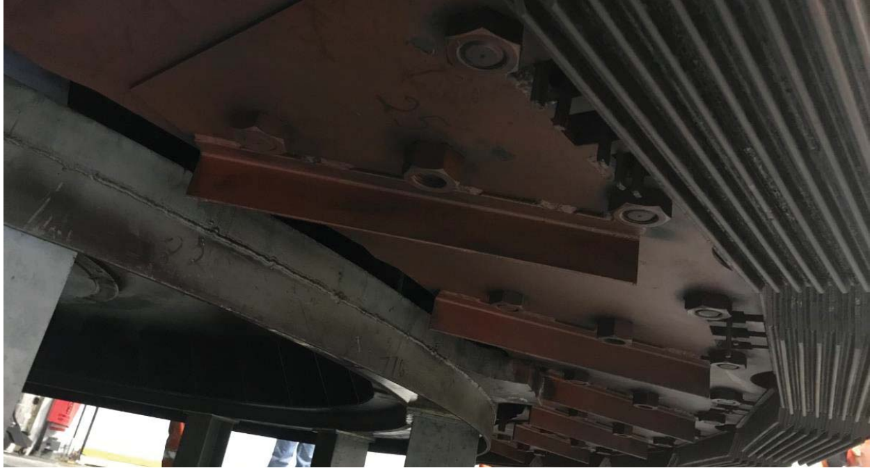
Figure 5-93: Rotor Rim, Bottom View 1
