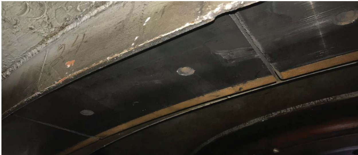
Figure 5-94: Rotor Rim, Bottom View 2 - Brake Ring
