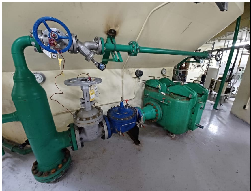
Photo 3: Line 2 Pressure Reducing Valve and Filter
