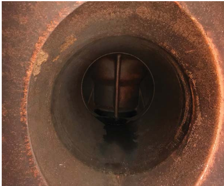
Figure 5-167: Spiral Case, Pressure Relief Valve
