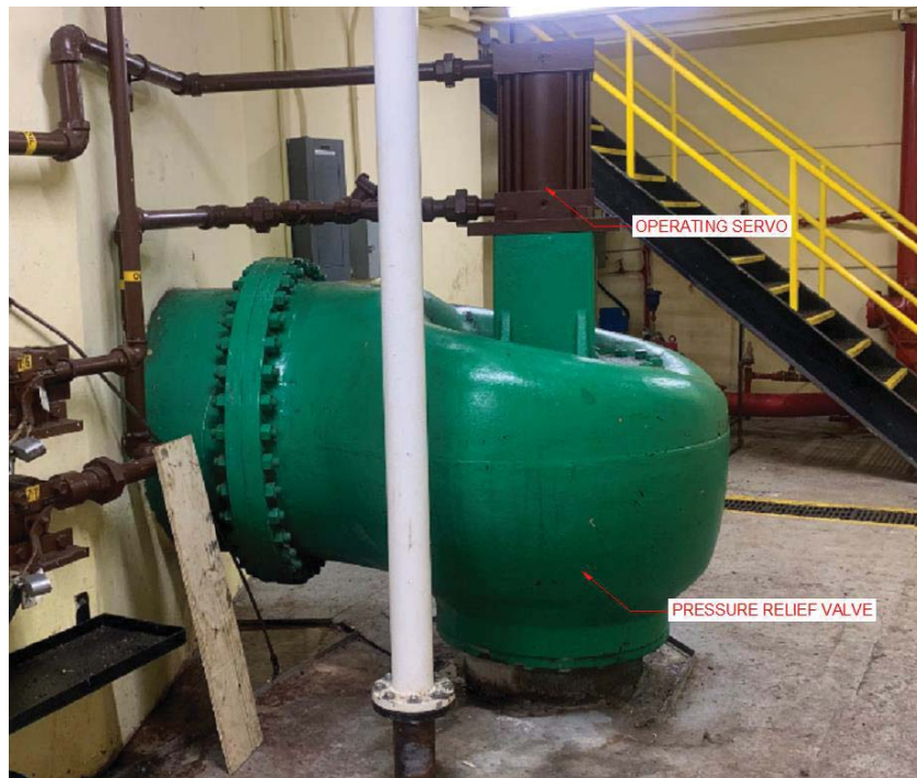
Figure 8-1: Pressure Relief Valve and Operating Servomotor
