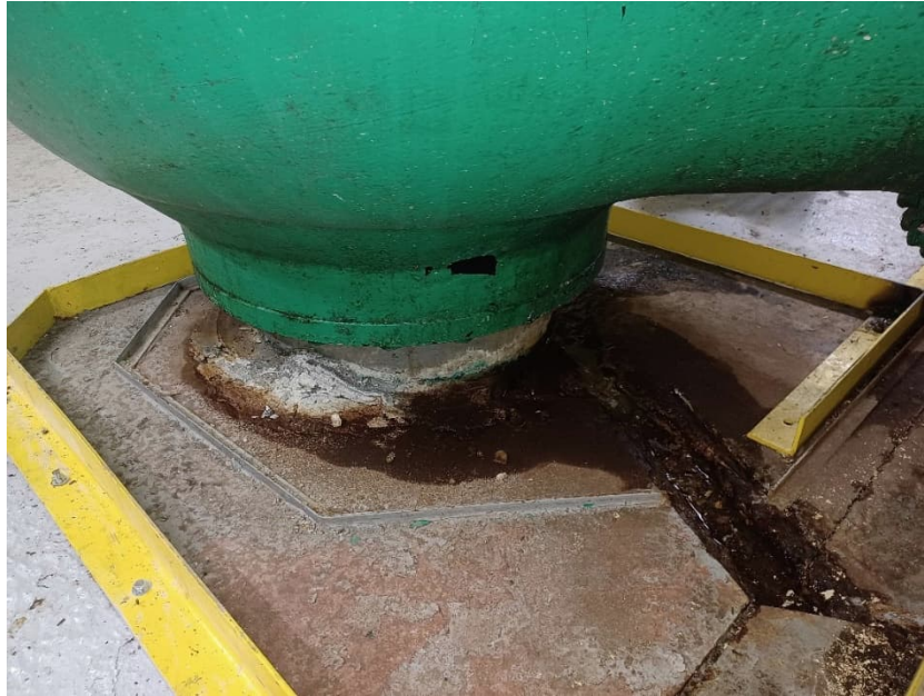
Figure 3-35: Relief Valve Discharge Pipe Leakage (Unit Dewatered)
