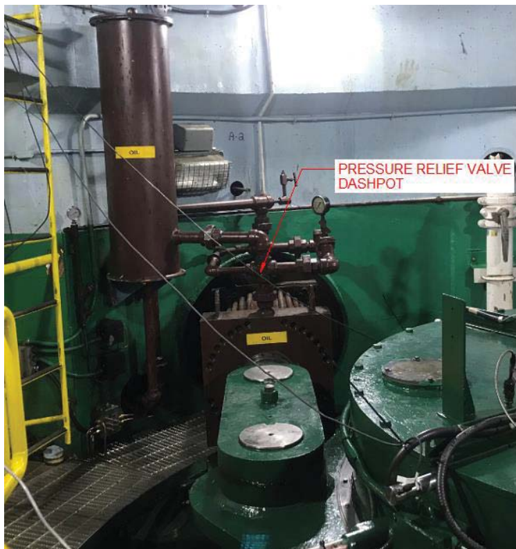
Figure 8-2: Pressure Relief Valve Dashpot
