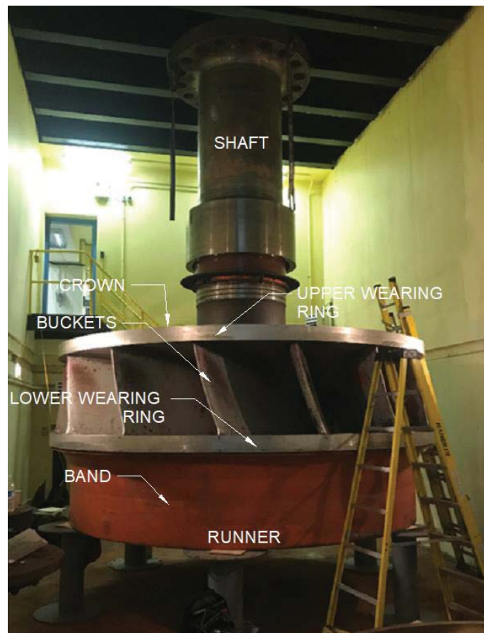
Figure 5-14: Turbine Runner Diagram
