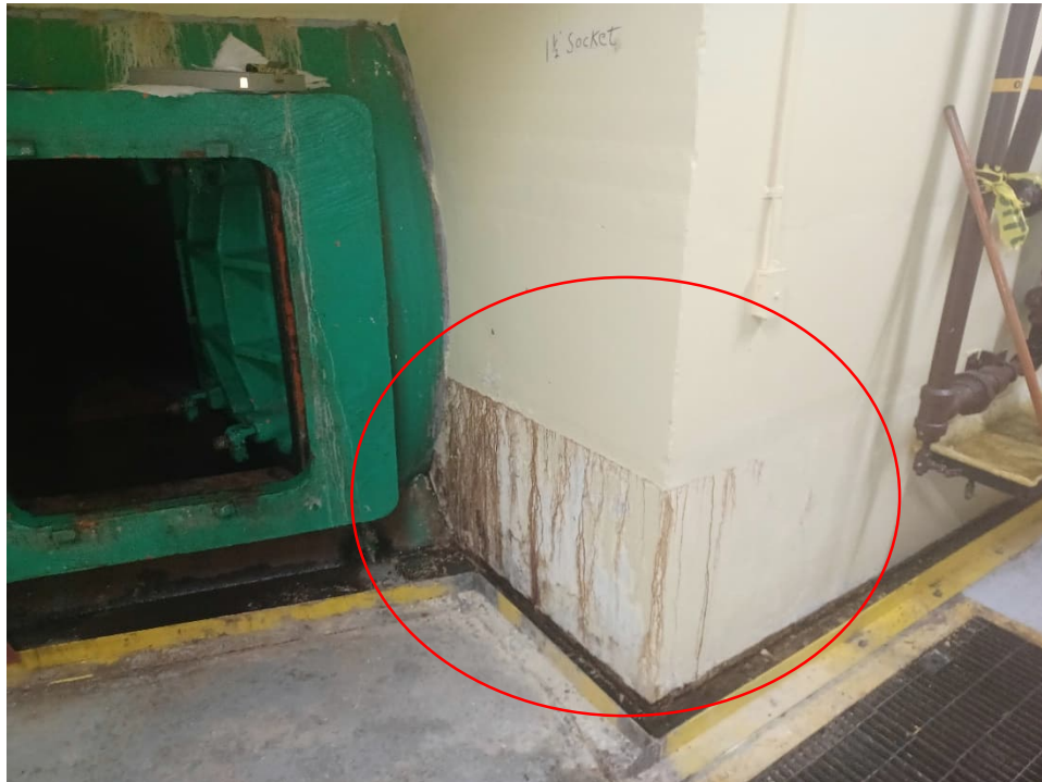
Figure 3-34: Water Seepage Between Concrete Pours
