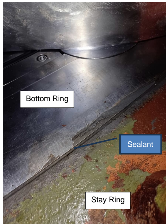
Figure 3-19: Silicon Sealant between Bottom Ring and Stay Ring (October 2023)
