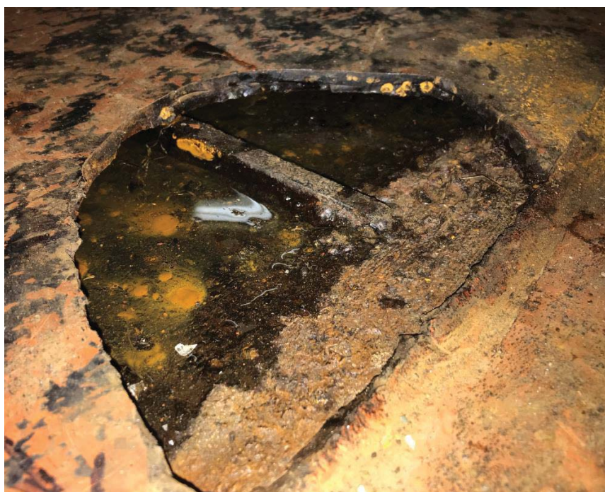
Figure 5-27: Balance Plate Missing Piece, VT-6
