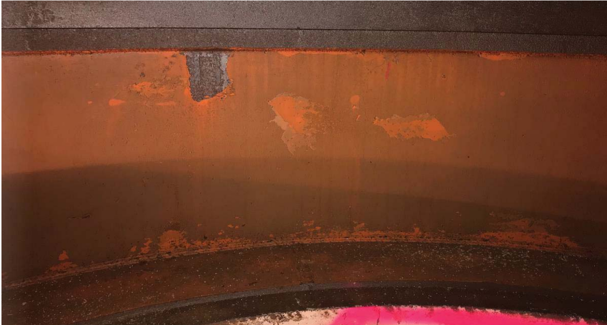
Figure 5-288: Discharge Ring, Paint Condition
