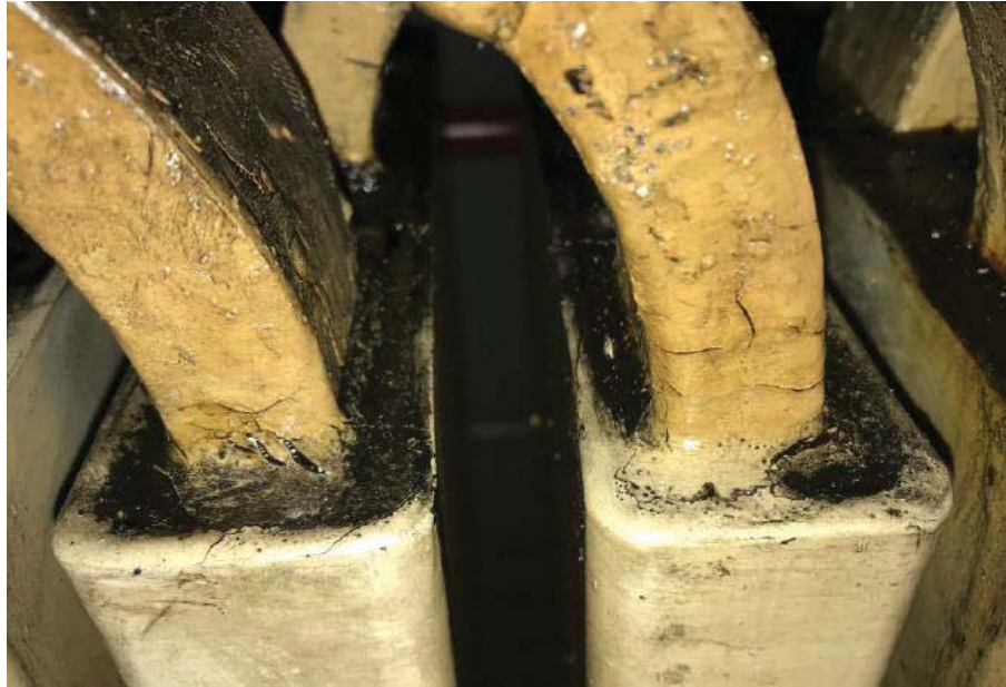
Figure 5-143: Stator Windings: Typical State of Lower End-Cap
