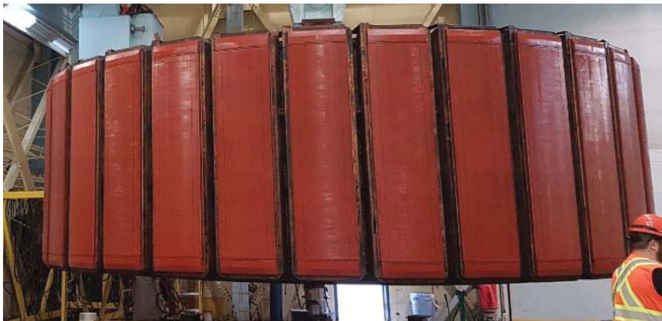
Figure 5-113: Unit 7 Rotor after Cleaning and Painting
