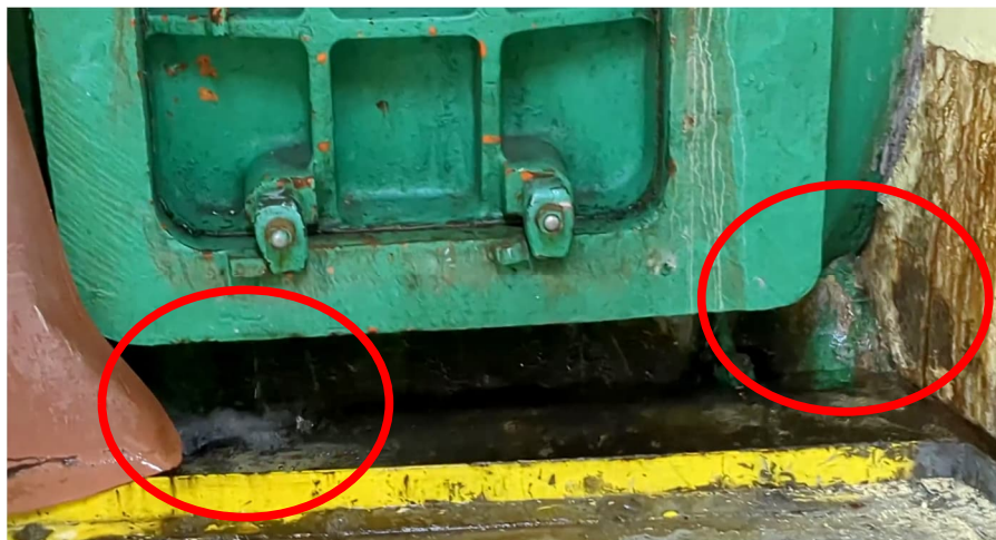
Figure 3-17: Scroll Case Leakage
