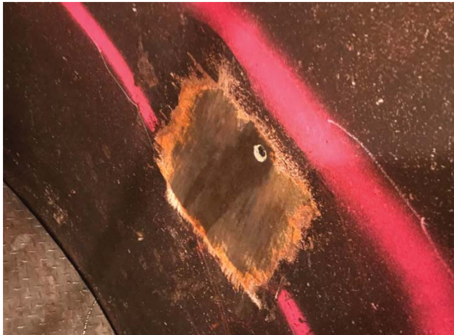
Figure 5-13: Draft Tube Void Mapping
