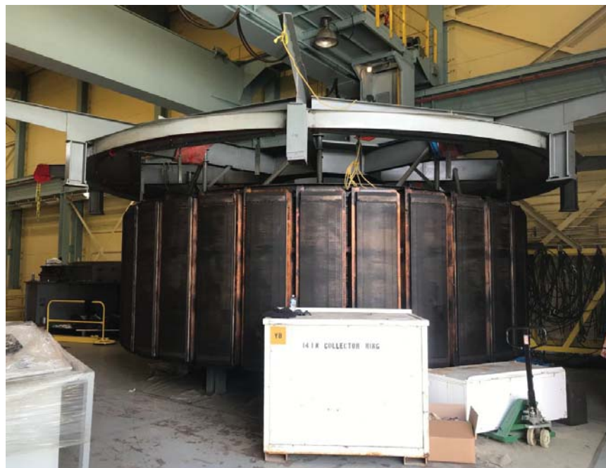
Figure 5-83: Rotor, Removed from Stator
