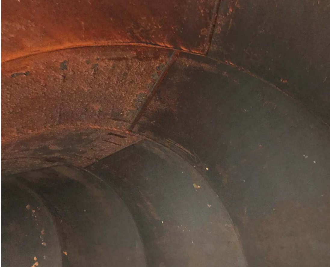
Figure 5-168: Spiral Case
