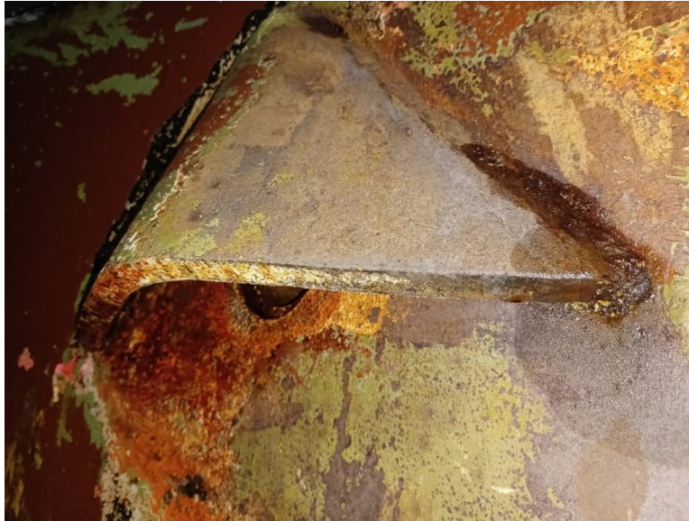
Figure 3-15: Aeration Pipe Injection Pipe to Draft Tube with Scoop / Cover
