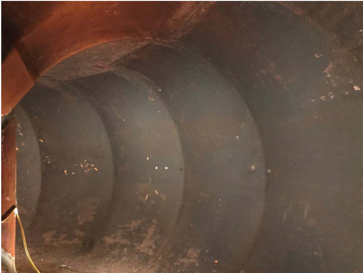
Figure 5-165: Spiral Case, Upstream
