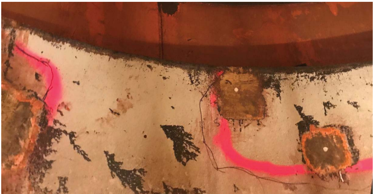
Figure 5-12: Draft Tube Void Mapping
