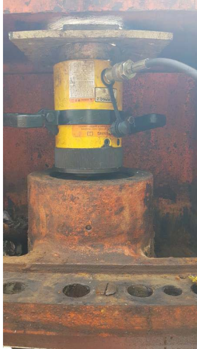
Figure 5-206: Head Cover, Intermediate Gate Stem Bushing Removal
