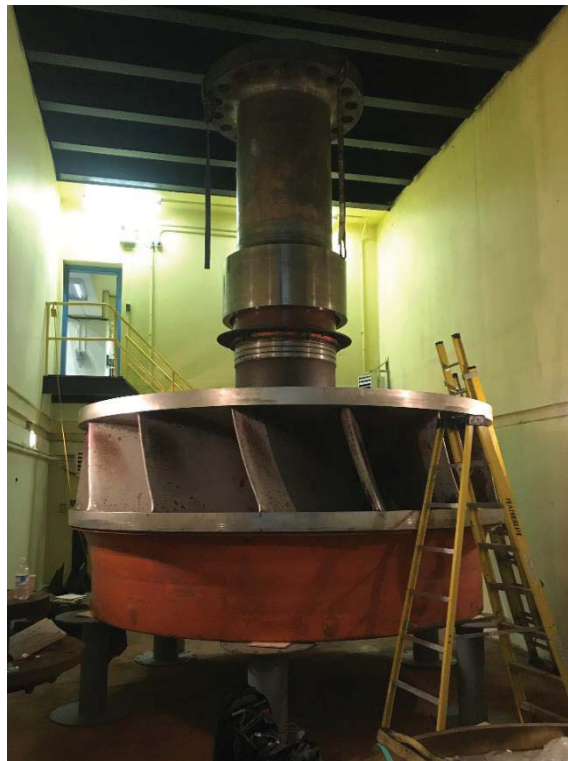
Figure 5-46: Turbine Shaft, Assembled to Runner
